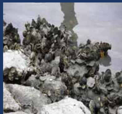
Rip-Rap Bay Structure with Oyster Growth
